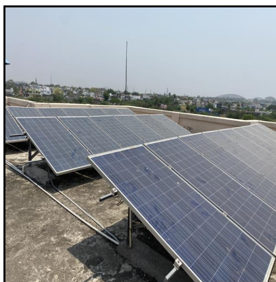
Figure: Solar Plant 8.90 KWp and Inverter System
