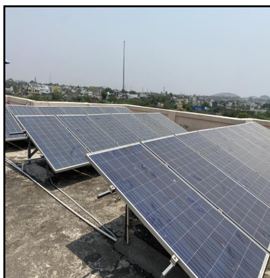
Figure: Solar Plant 8.90 KWp and Inverter System
